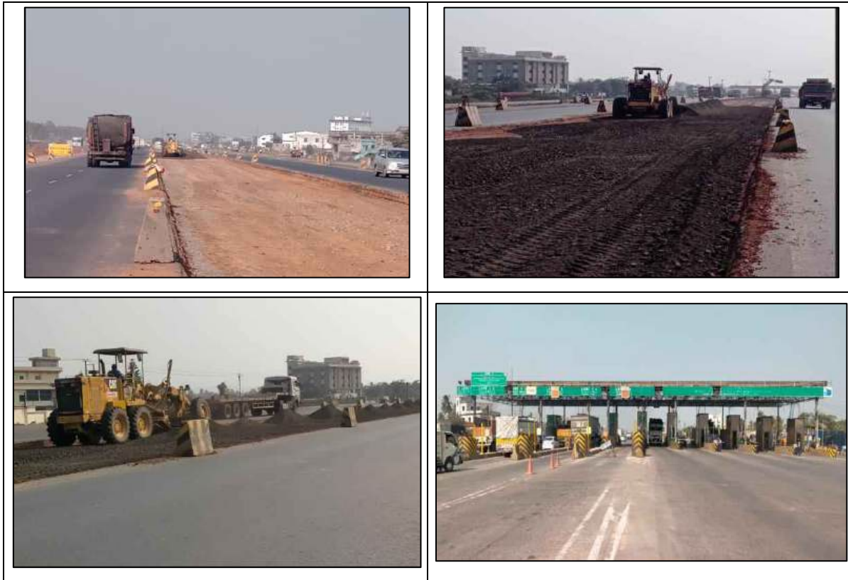
Figure 2-2: Photographs showing Project Corridor
