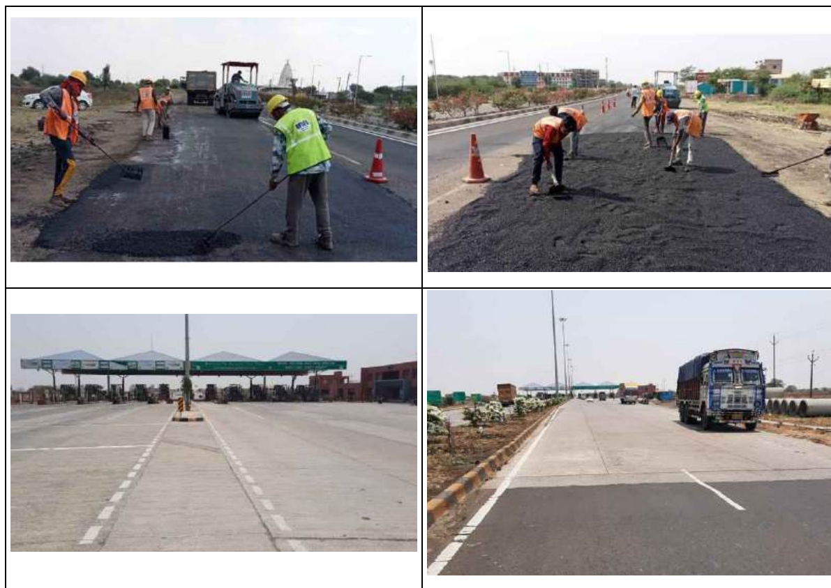
Figure 2-2 : Photographs showing Project Corridor
