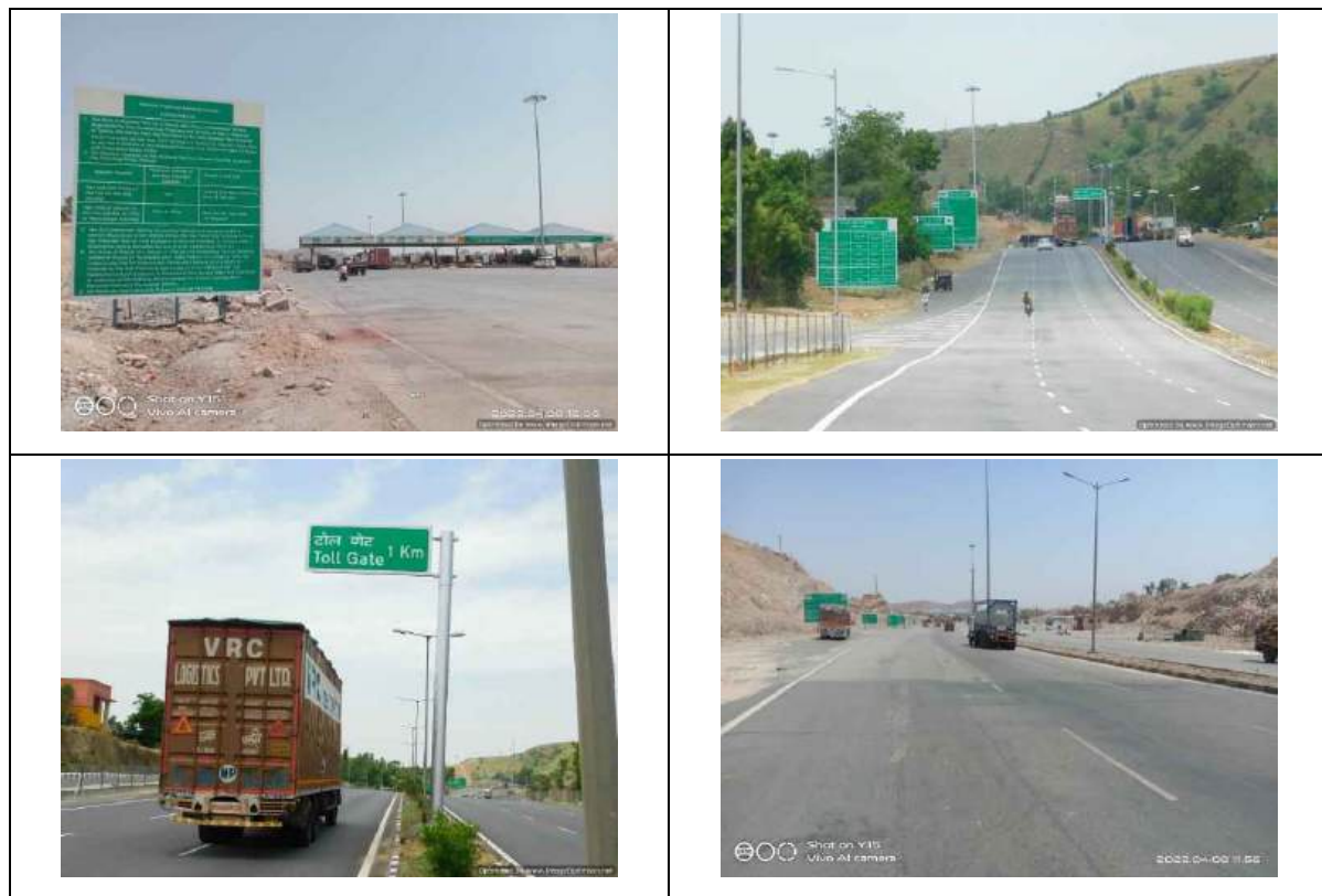
Figure 2-2 : Photographs showing Project Corridor
