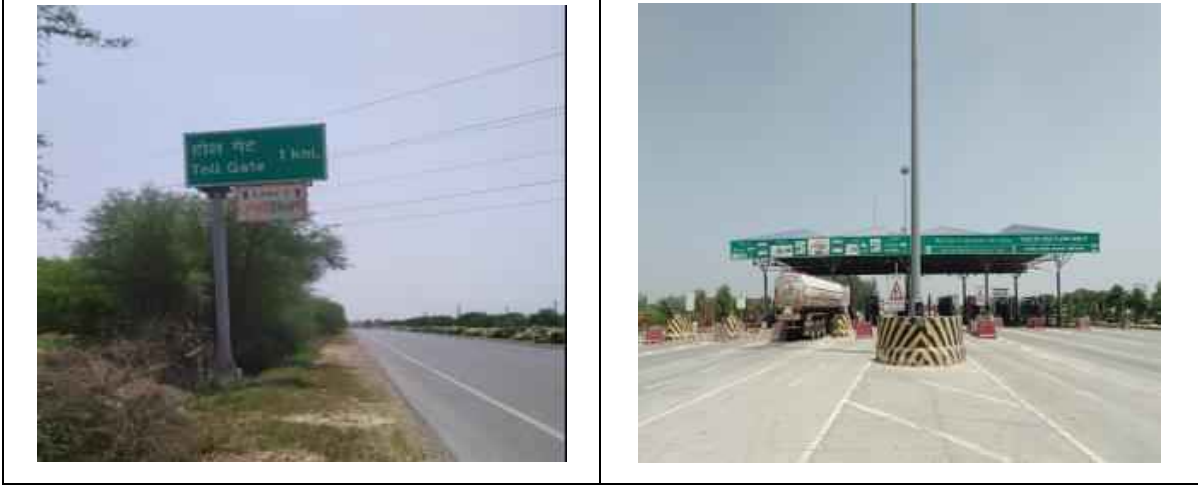
Figure 2-2 : Photographs showing Project Corridor
