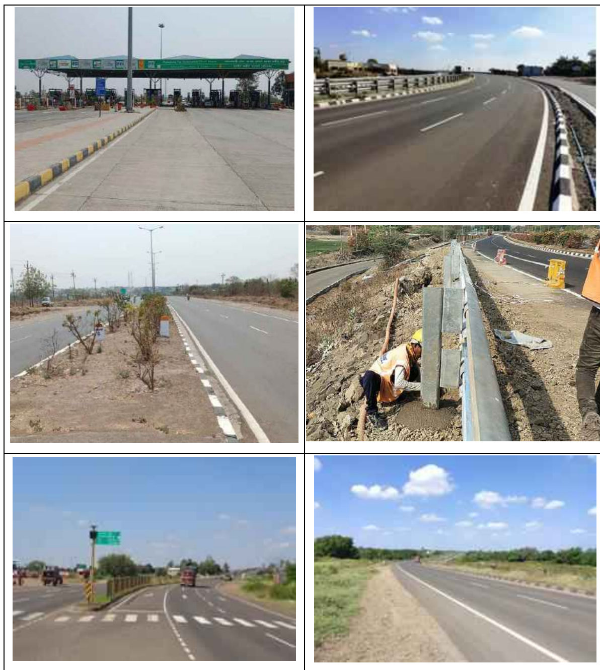
Figure 2-2: Photographs showing Project Corridor
