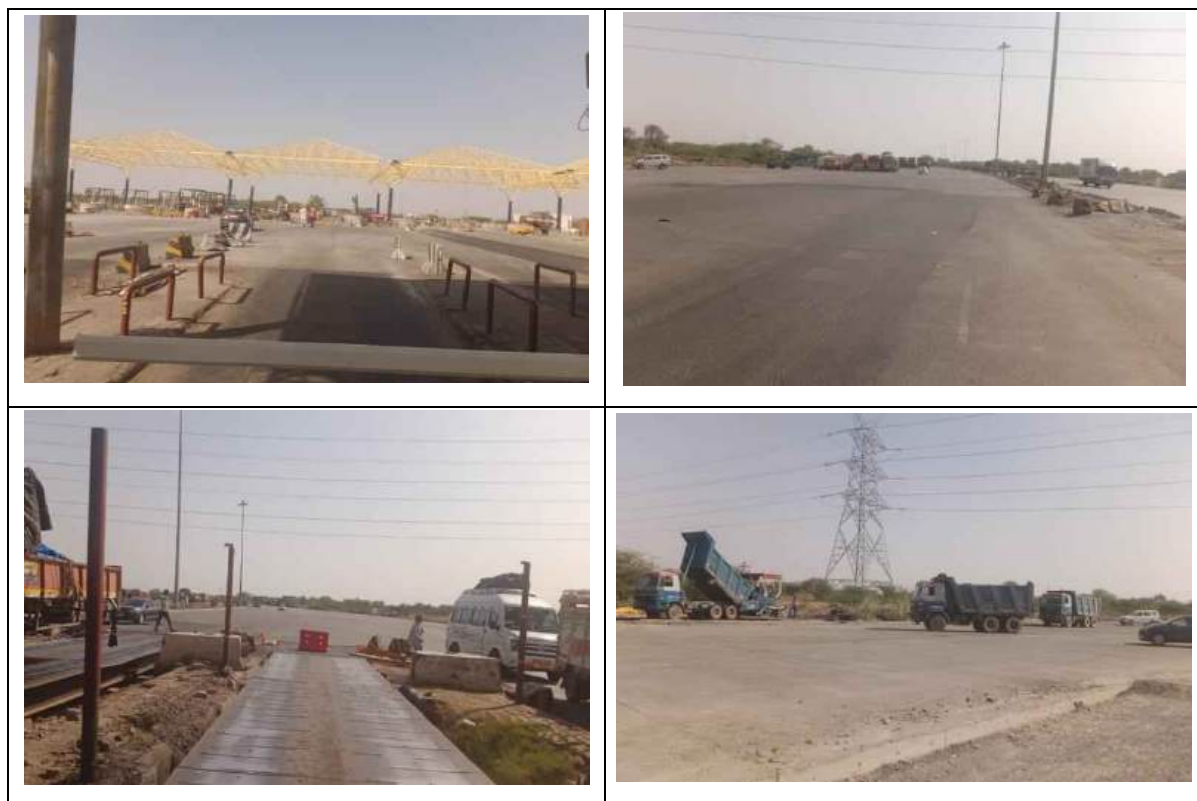
Figure 2-2 : Photographs showing Project Corridor
