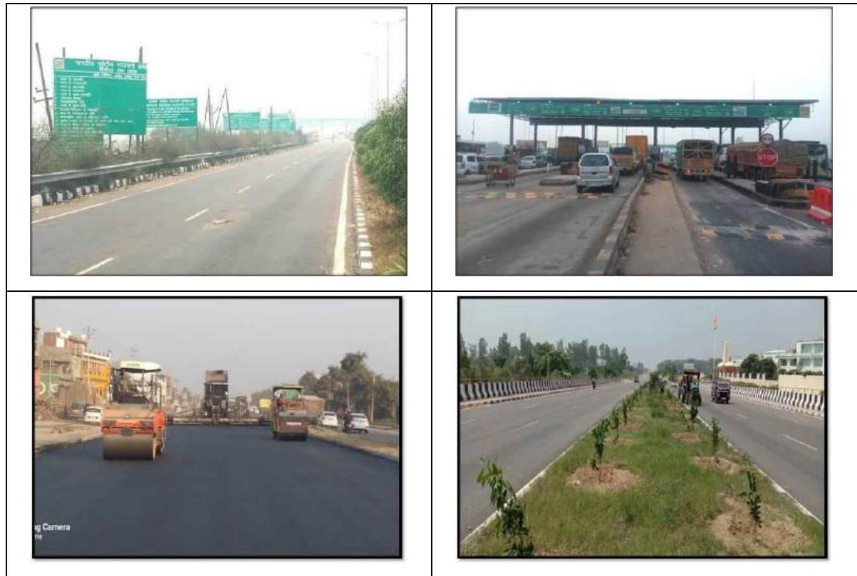
Figure 2-2: Photographs showing Project Corridor
