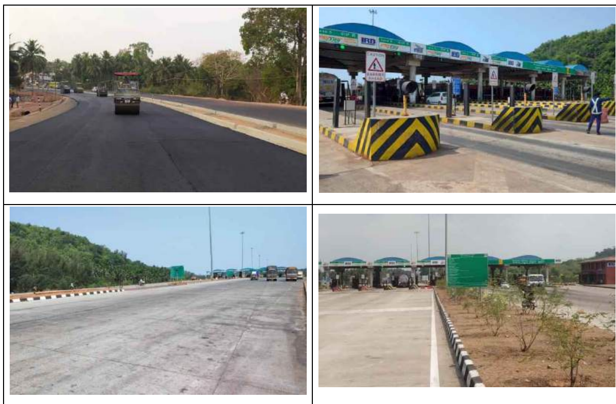
Figure 2-2 : Photographs showing Project Corridor
