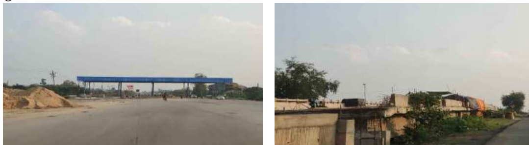
Figure 4-5 ROB & Toll Plaza under construction.
